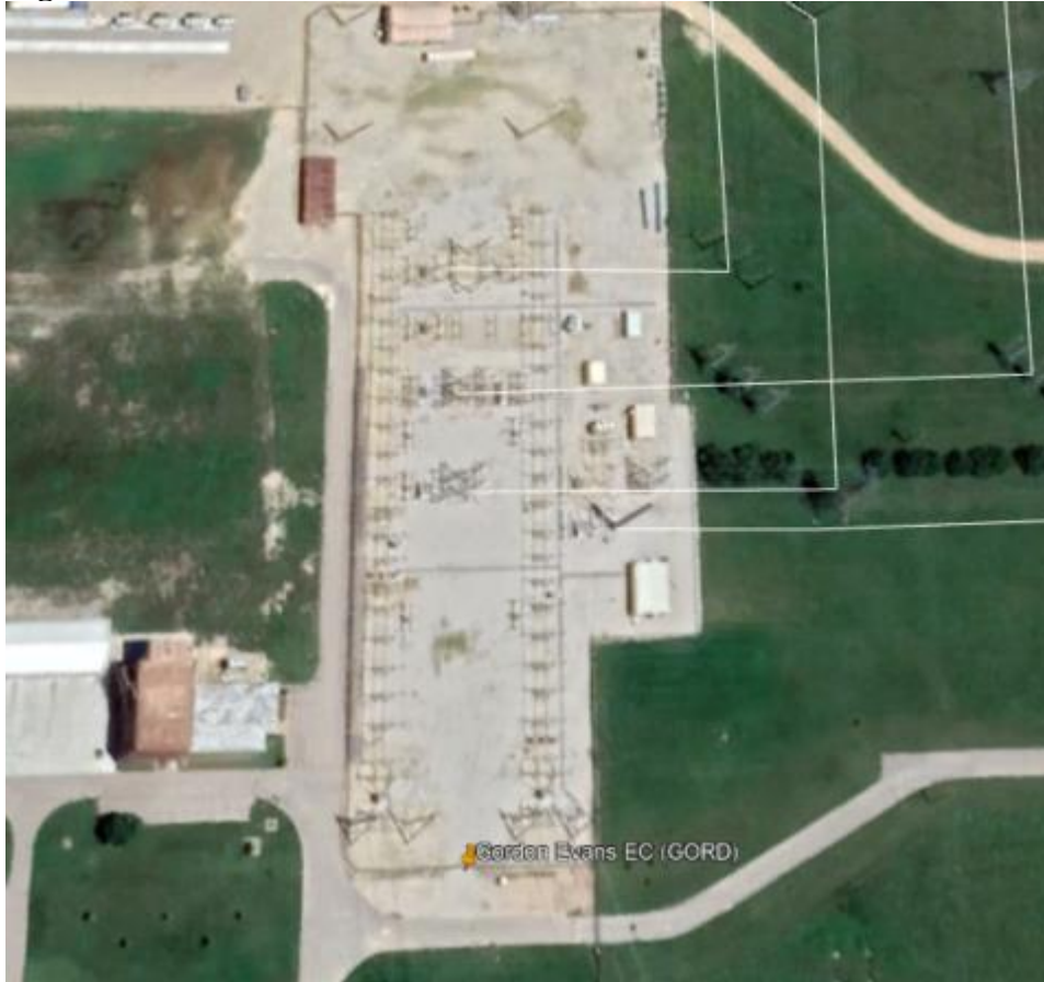
Figure 33 – Gordon Evans 138kV Substation
